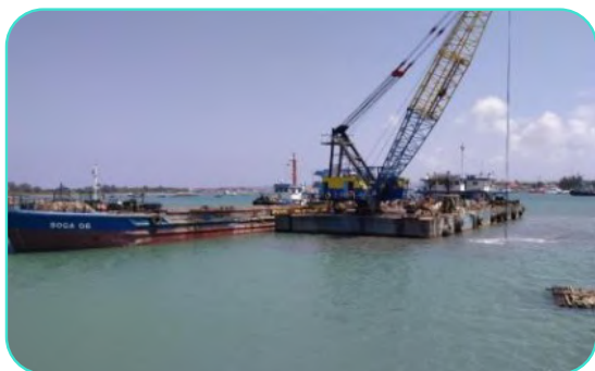
Gambar Pengerjaan Pengerukan Paket A Picture of Dredging Work in Package A
