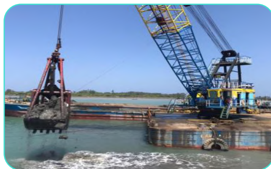
Gambar Pengerjaan Pengerukan Paket A Picture of Dredging Work in Package A
